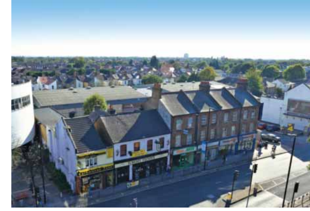
ACTUAL FOURTH FLOOR VIEWS LOOKING SOUTH
