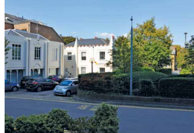
ACTUAL GROUND FLOOR VIEWS LOOKING NORTH
