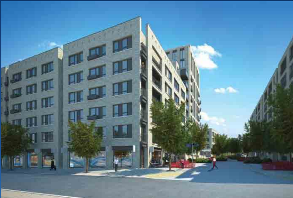
Canary Point looking towards the development's Home Zone
