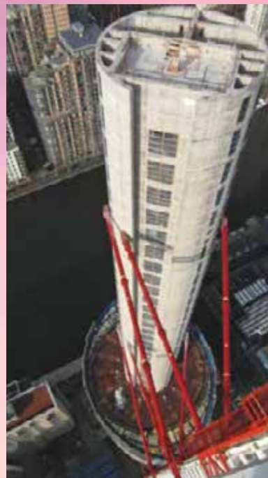
Core construction January 2015
