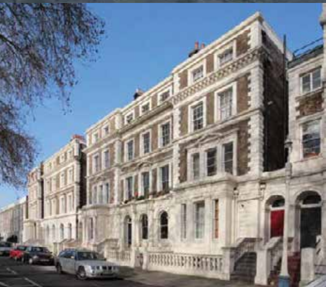
A conservation area terrace, Stockwell
